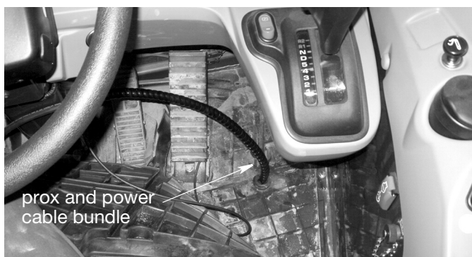
FIG. 62: View inside cab under floor mat
